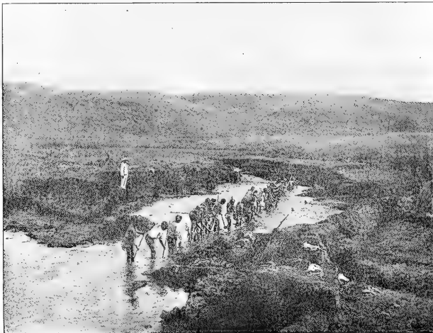
Method of getting rid of earth by deflecting stream through diggings at end of day. Nearer view of lava-stream beyond the marsh.
